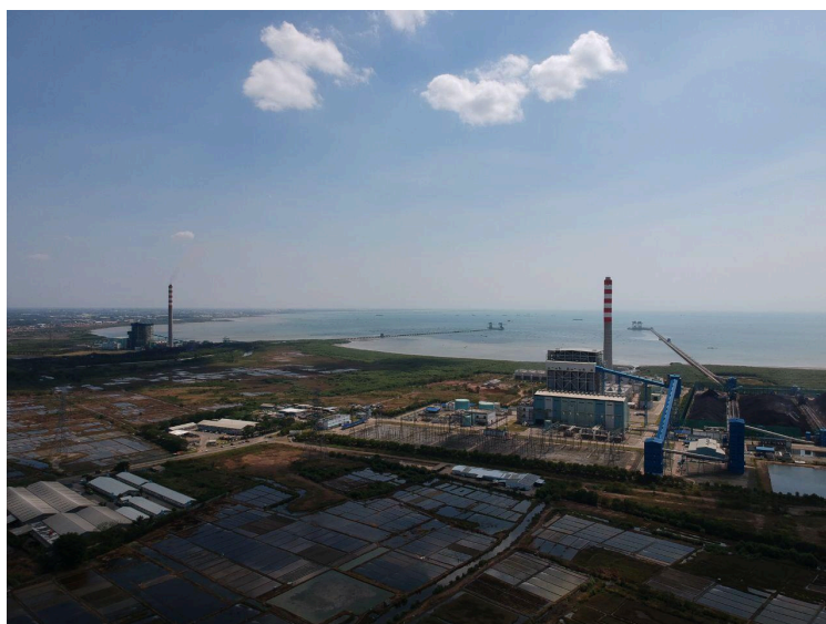
Photo: Cirebon-1 coal-fired power plant (in the back), which has been in operation since 2012, and Cirebon-2 that started the operation in May 2023 (Indonesian Forum for the Environment (WALHI) West Java, June 2023)
