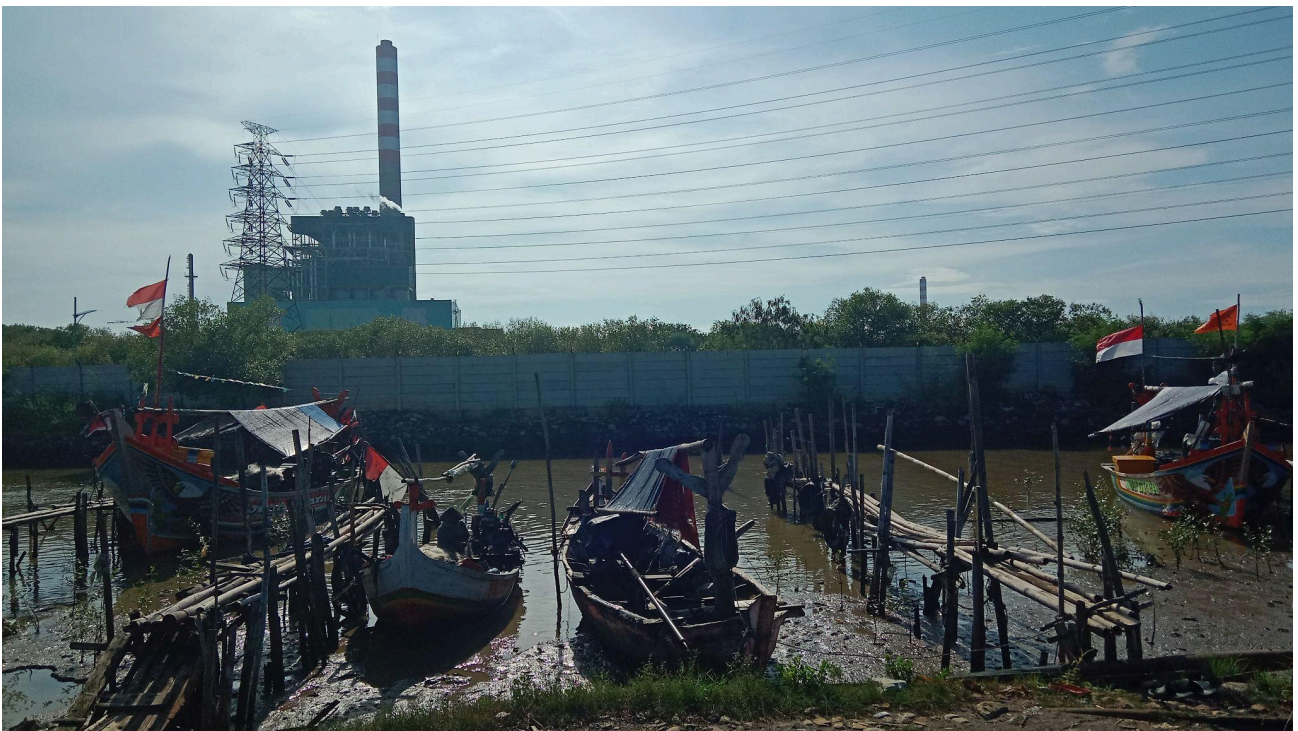
Photo: Fishing port where fishing boats of Waruduwur village are anchored and the Cirebon-1 coal-fired power plant which has been in operation since 2012 (FoE Japan, April 2024)
