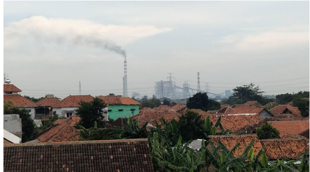
Photo: Unit 2 (adjacent to Unit 1) is currently under trial operation (FoE Japan, Nov. 2022)
