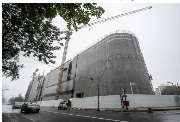
Y Complex Project Construction under way (2021)
