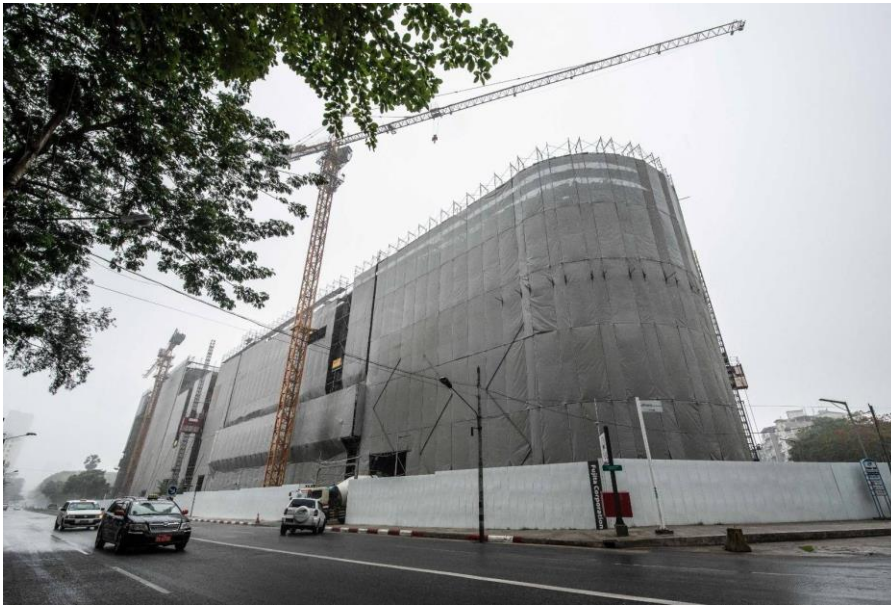
Figure 2: Y Complex under construction (2021. Photo credit: Myanmar Now)
